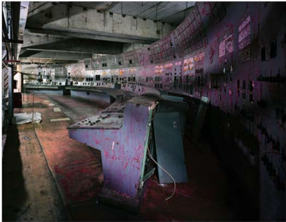
Control Room, Reactor 4, Chernobyl, 2001.
