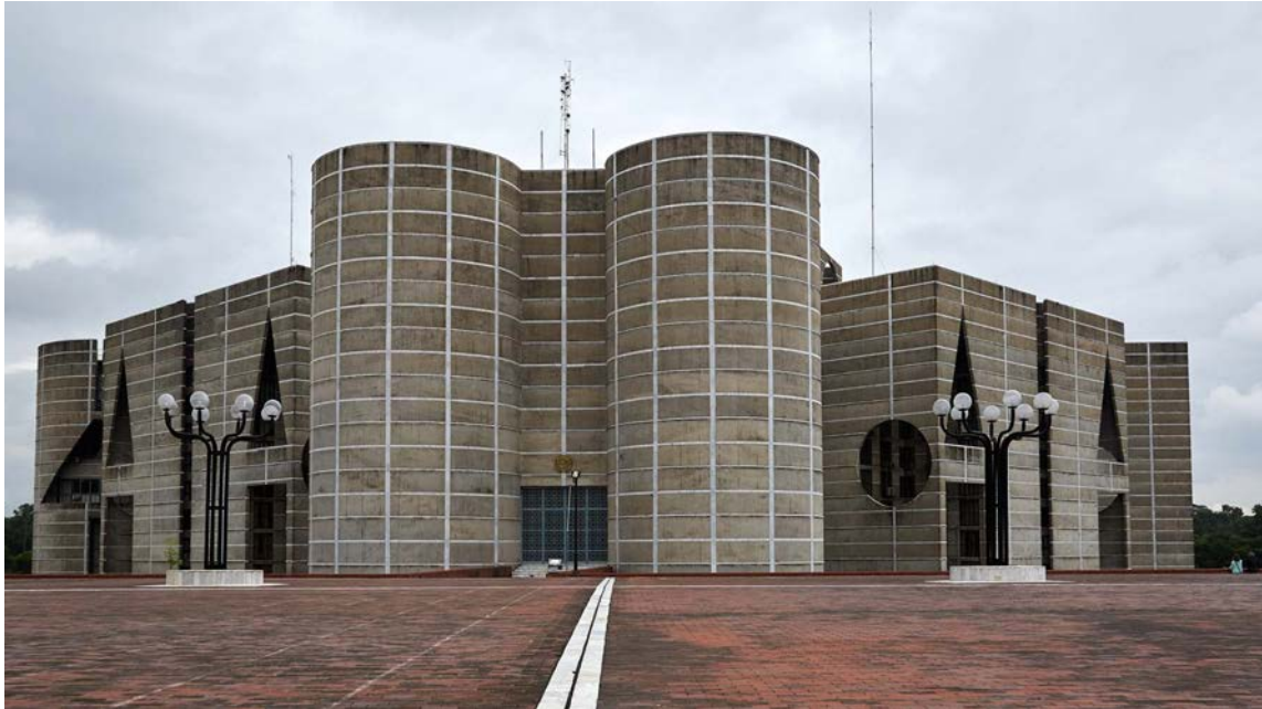
National Parliament House located at Sher-e-Bangla Nagar in Dhaka, Bangladesh was designed by architect Louis Kahn
