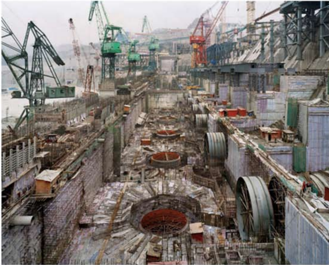
"Dam #6," Three Gorges Dam Project, Yangtze River, 2005. (Edward Burtynsky)
