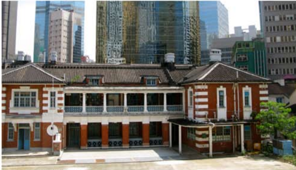
Photo by Isabelle de Wavrin, 2011 The Central Police Station, Central Magistracy and Victoria Prison compound will be transformed into an art museum.
